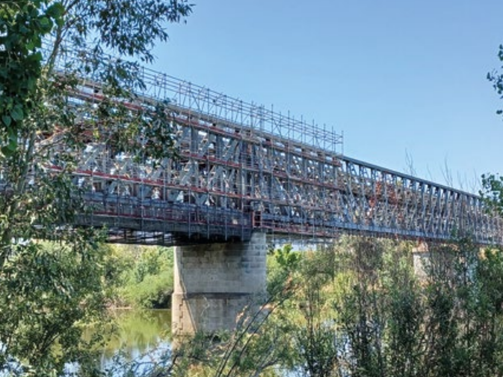
◀ Maintenance and reinforcement of the Guadiana river metal bridge (Mérida)
