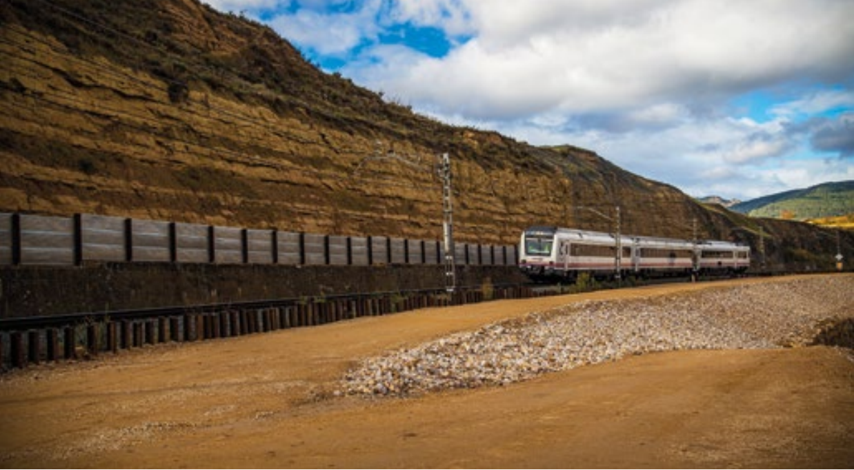
△ Stabilisation of earthworks in Castejón de Ebro-Bilbao line (La Rioja)
